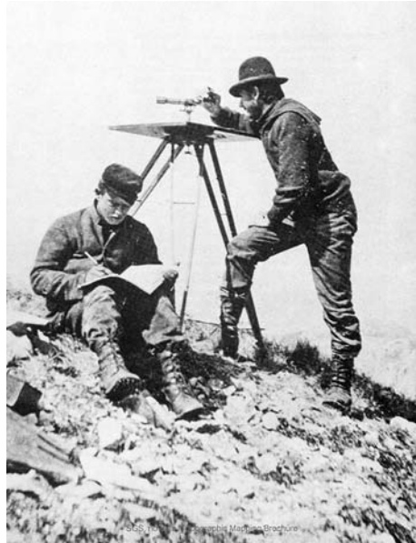
FIGURE 7.2. Surveyors at work with a plane table. From http://erg.usgs.gov/isb/pubs/booklets/topo/topo.html
